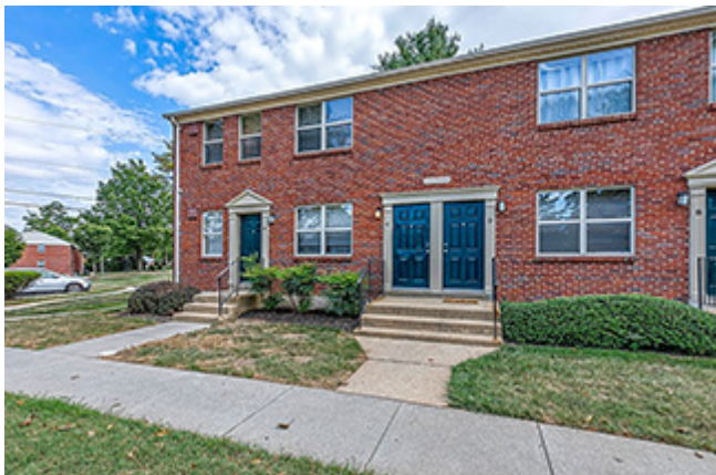
One of the many apartment complexes that Pressley Ridge-New Pathways utilizes for the Independence Plus Program.
